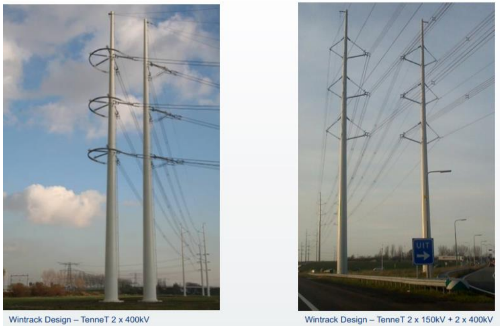
Figure 1: New 400 kV monopole designs in the Netherlands
